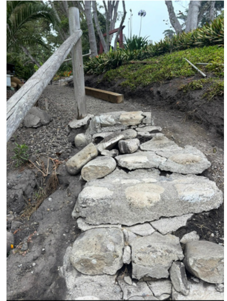
Beach Stairs Before
