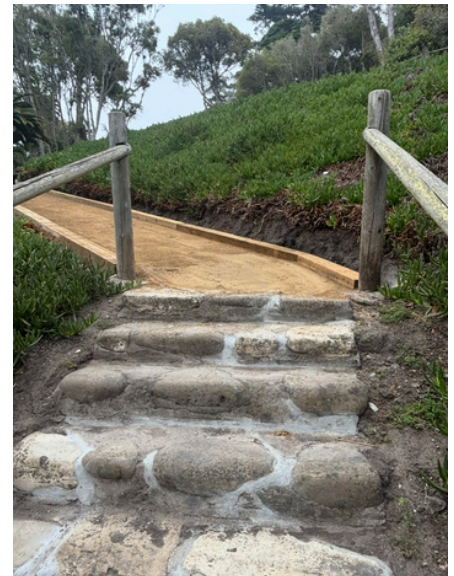
Beach Stairs After
